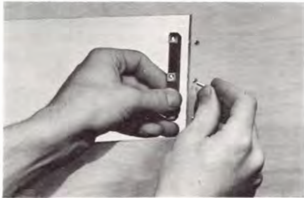
Figure 20. Securing Mounting Strips to Installation Cutout.
