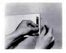
Secure the mounting strips to the rear of the cabinet panel using two screws from the hardware package.
