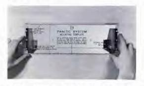
Place the template over the mounting screws. The mounting screws should be centered in the "A" and "B" holes on the template. The sides of the mounting brackets should match the vertical dash lines on the template. If necessary, loosen the screws and push the brackets into alignment and retighten.
